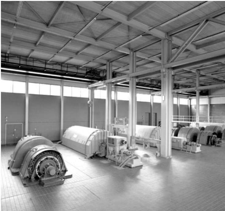
Figure 10.4 Two of the four short-circuit generators with their auxiliary machines in KEMA's generator room (courtesy of KEMA)
