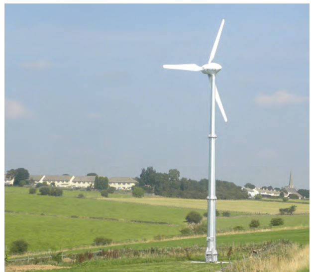
Photo courtesy of Evoko Energy Ltd
