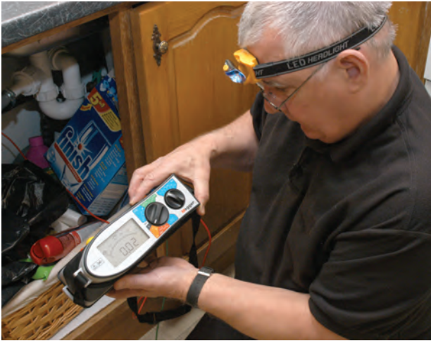
A continuity test being carried out
