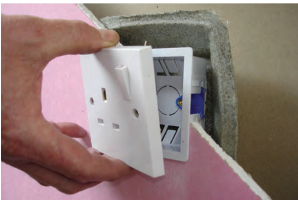
Fire and acoustic rated cover fitted behind a dry lining box (Photo courtesy of Tenmat Ltd)
