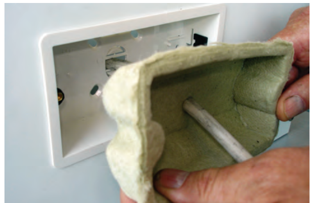
Intumescent insert being installed in a dry lining box (Photo courtesy of Tenmat Ltd)
