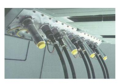
Figure C-30: Examples of plug-in surge arresters
